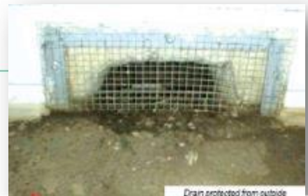
Drain protected from outside
